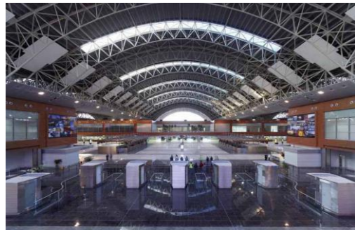
Sabiha Gokcen International Airport is one of the world's most earthquake-proof buildings.
